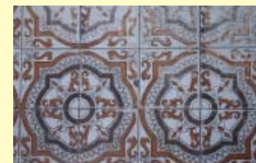
Piso do hall principal
