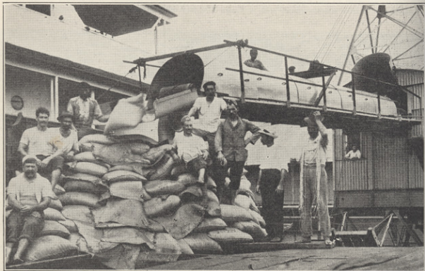
DELIVERY END OF THE ENDLESS RUBBER CONVEYOR OVER THE SHIP'S HOLD
